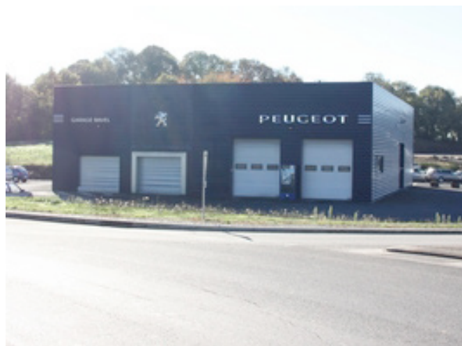
Garage automobiles RAVEL
